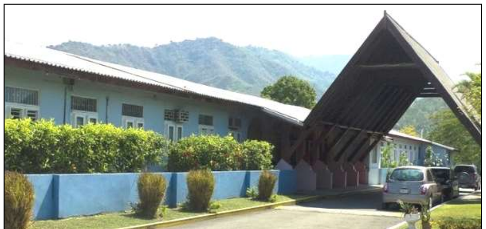
One of the structures on the UTCWI campus, located in Kingston, Jamaica
