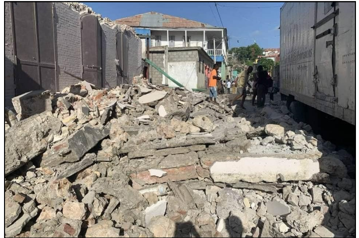
The images above and below show some of the destruction that resulted from the August 14 earthquake.
